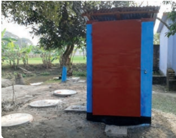
Above: Under construction in Satkhira - a twin-pit raised step toilet.
